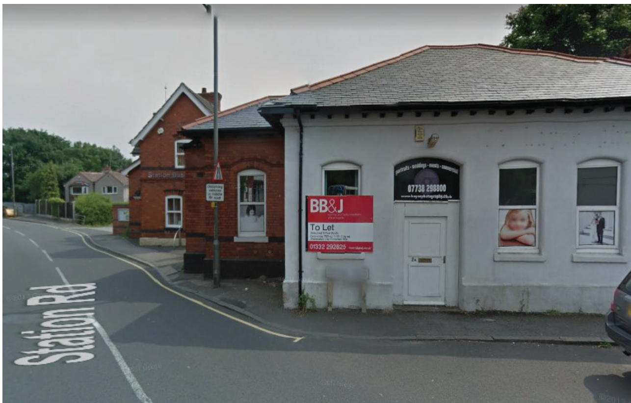
Figure 5: Pedestrian Pinch Point, Station Road (Taken from Google Maps 2018)
